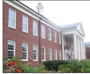
University of North Carolina at Wilmington, North Carolina
